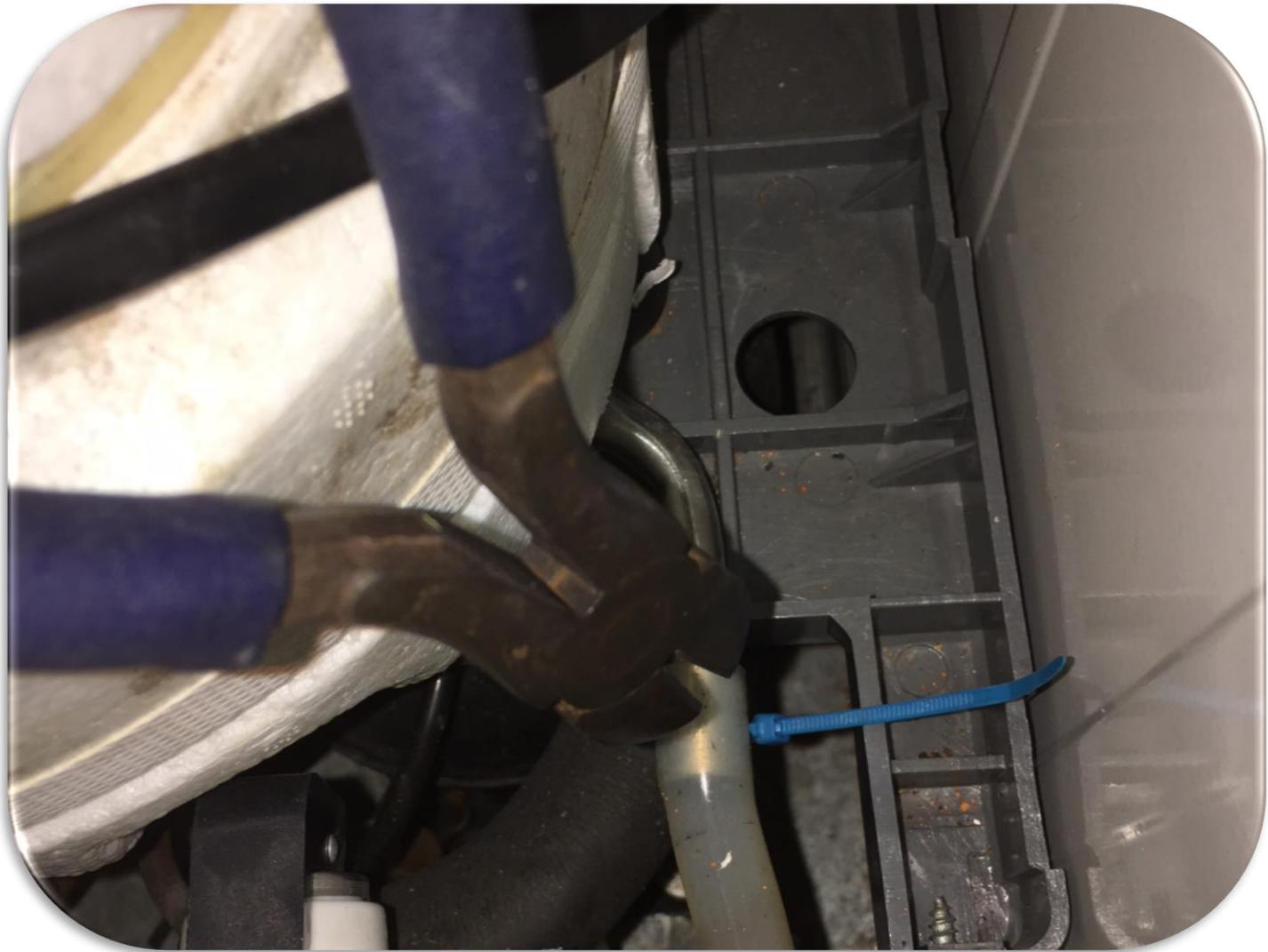
Cut off zip ties that secures silicone pipes to steel pipes
