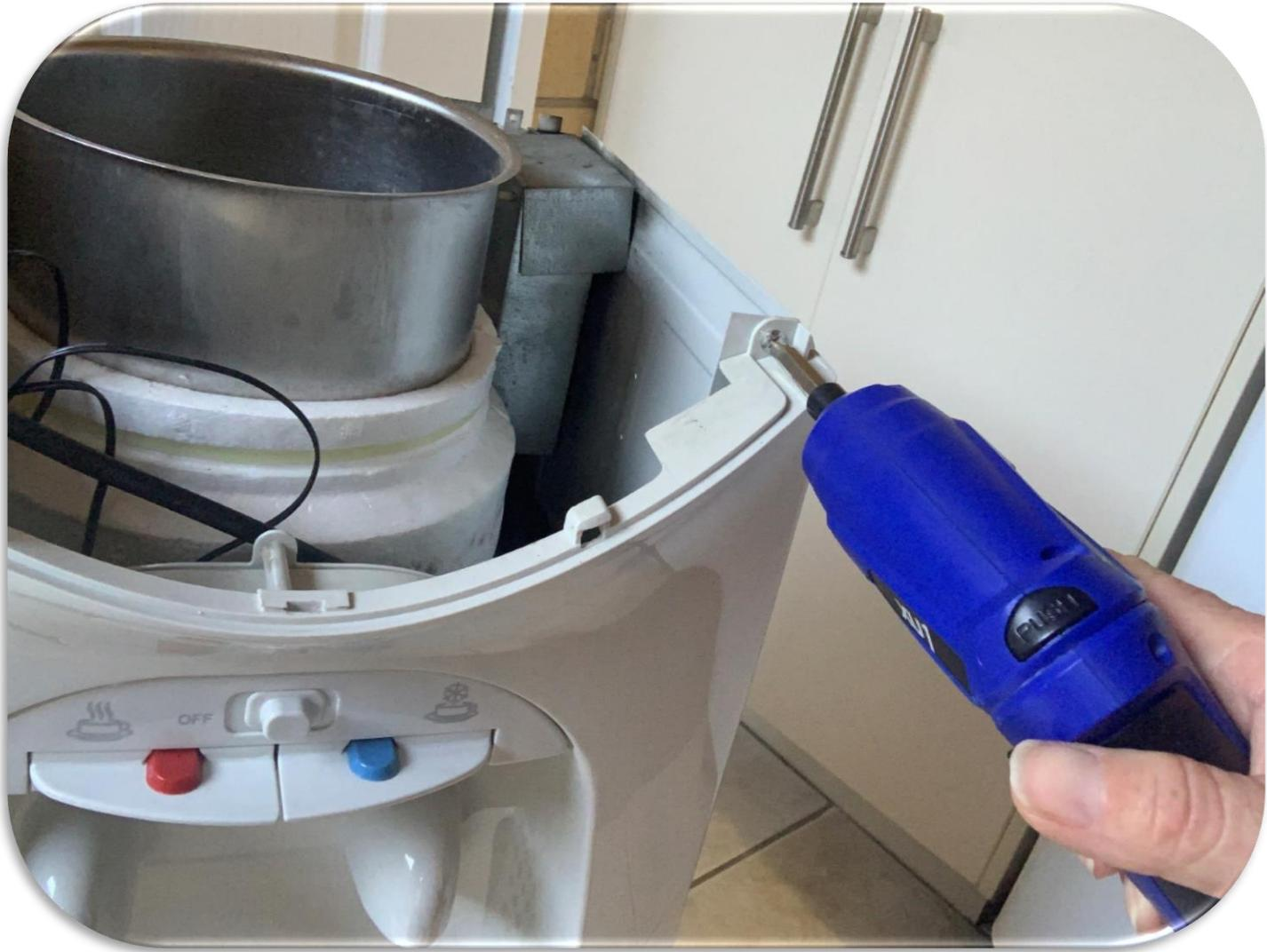
Remove 2 x screws at the front once lid has been removed.
