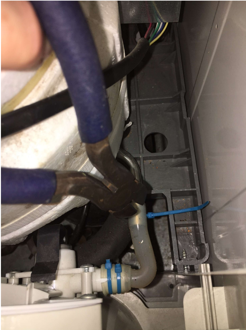
5. Cut zip tie securing silicon tube to pipe
