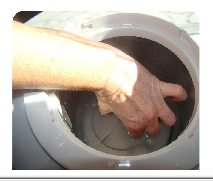
Pull out plastic base plate by putting fingers through holes and pull it straight up, might to give it a few twists to get it to come out.
