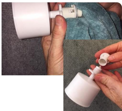
Hold on to the nut on the inside of the bowl and unscrew anti clockwise to undo the bottom part of float valve. You might need to use a tea towel to get a grip
